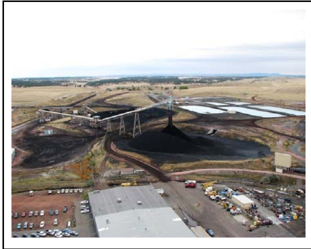
ETIC Tour of Colstrip Steam Electric Station, October 2007. Photo courtesy of Lindsey Waggoner, outreach coordinator, Big Sky Carbon Sequestration Partnership.
