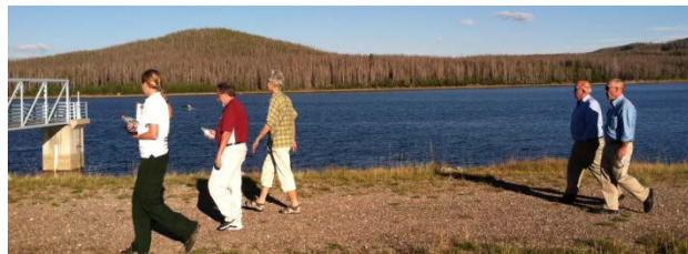
Chessman Reservoir is the primary drinking water source for the City of Helena.
