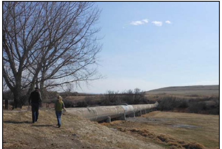
Fort Shaw Irrigation District Siphon Repair Renewable Resource Project Grant
