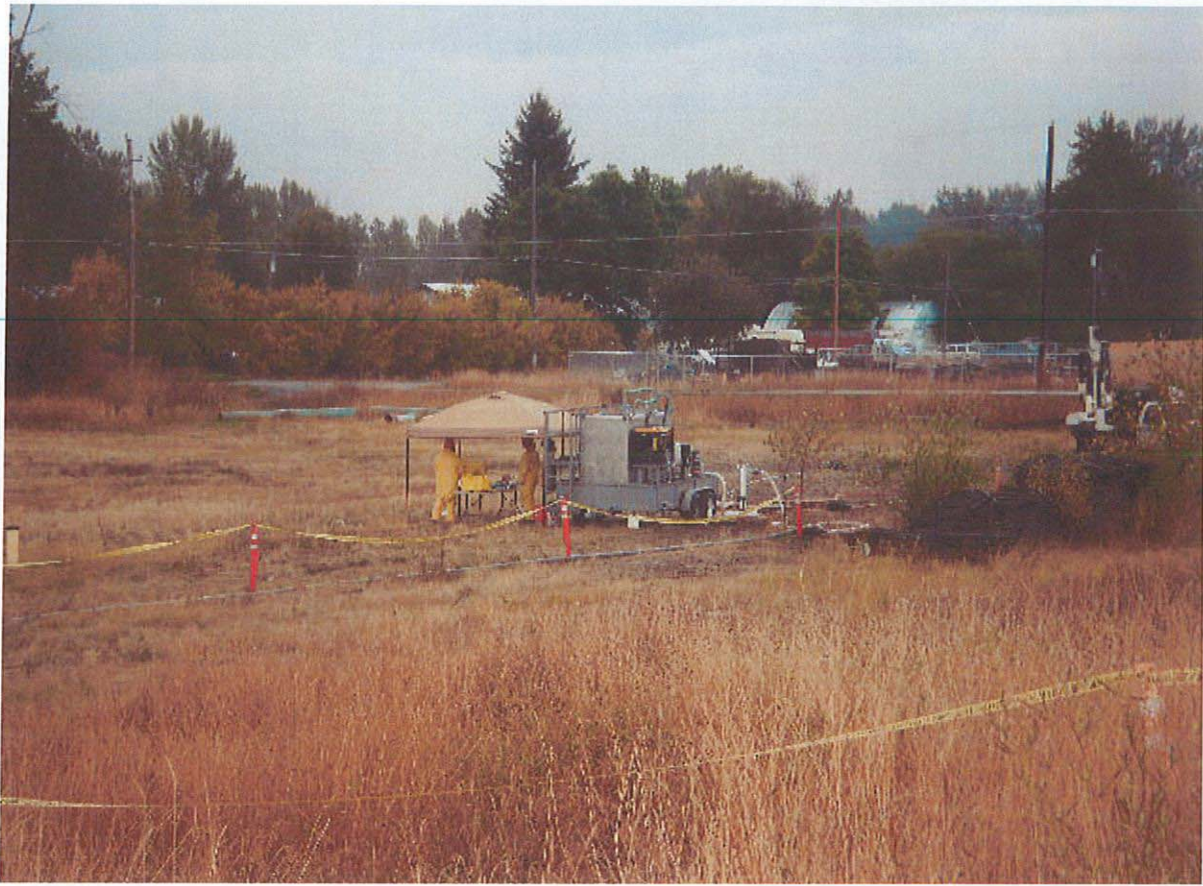
Photo 7: 10/5/11 - BNSF contractors performing chemical oxidation injections at the KRY Site.
