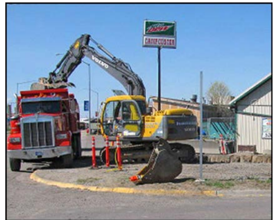
Excavating petroleum contaminated soil, Hardin (April 2016)
