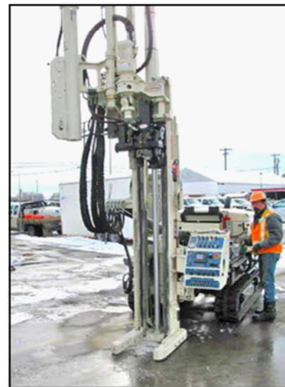
Installing soil boring at a former service station, Billings (January 2016)
