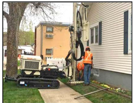
Testing soil for petroleum near residence, Lewistown (May 2016)
