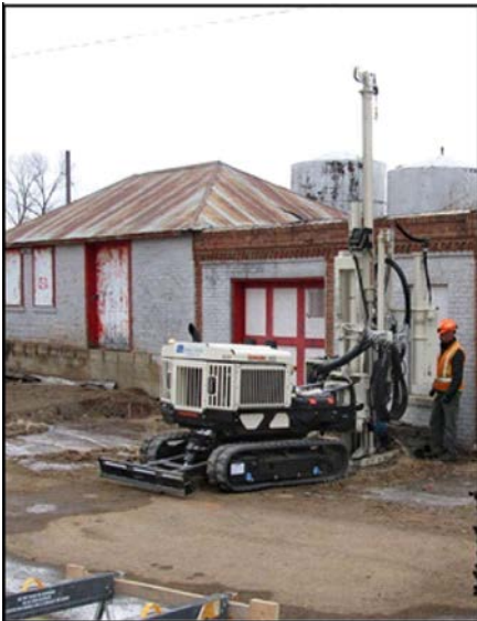
Installing borings at former service station, Plevna (February 2016)
