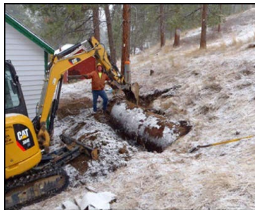
Removing half-buried tank at Unionville School (March 2016)
