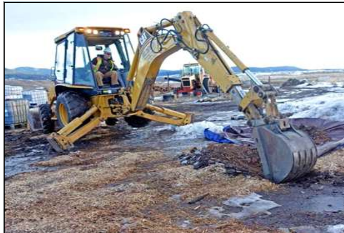
Removing hazardous waste at former wood treating facility, Lewistown (February 2016)
