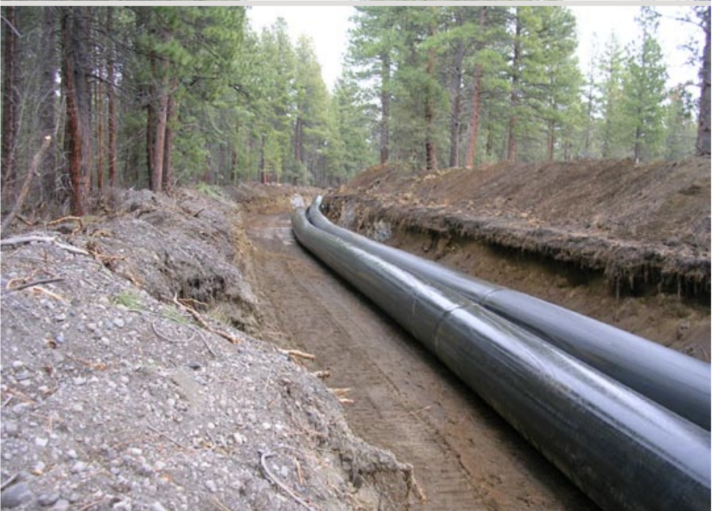
The Deschutes River Conservancy's water conservation project with the Three Sisters Irrigation District piped 3.8 mile section of their main canal located near Whychus Creek in Sisters, Oregon. Piping this section reduces water loss from leaking canal beds and enables the irrigation district to leave 6 cfs (3.8 million gallons of water per day) instream during the irrigation season. Photo courtesy of the Deschutes River Conservancy.
