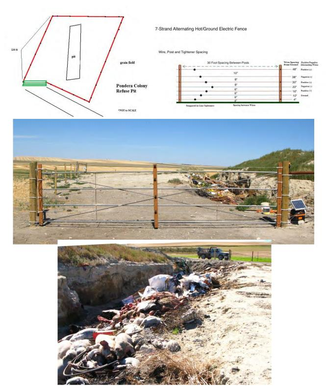
Figure 1. Design and completion of a permanent solar-powered electric fence system to prevent grizzly bear access to the Pondera Colony refuse site, 8/21/2013.
