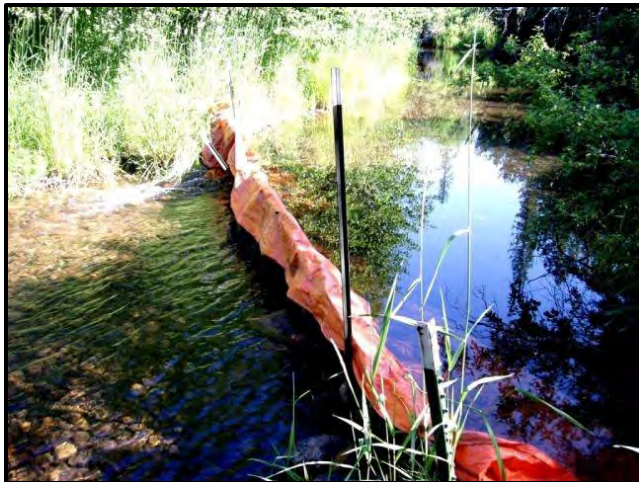
Photo Illustration 4. Fish screens installed on irrigation diversions located on Morrell Creek and Ninemile creeks. Morrell Creek, a tributary to the Clearwater River located near the town of Seeley Lake, supports an important fluvial bull trout population. The Morrell Creek project (upper photograph) involved reducing entrainment into two irrigation canals by installing fish screens, improving upstream fish passage, reducing periodic channel disturbance and enhancing instream flow while continuing to meet the needs of the water user. Ninemile Creek is a tributary to the Clark Fork River located near the community of Ninemile that supports westslope cutthroat trout, rainbow trout, brown trout and mountain whitefish. The Ninemile Creek project involved installation of a coanda style fish screen to prevent entrainment into the irrigation canal and installation of a vortex rock weir to enhance upstream fish passage while meeting the needs of the water user. The lower left photograph shows the Ninemile Creek diversion before project completion. The lower right photograph shows the installed coanda fish screen and vortex rock weir. All photos courtesy of Ladd Knotek, FWP.
