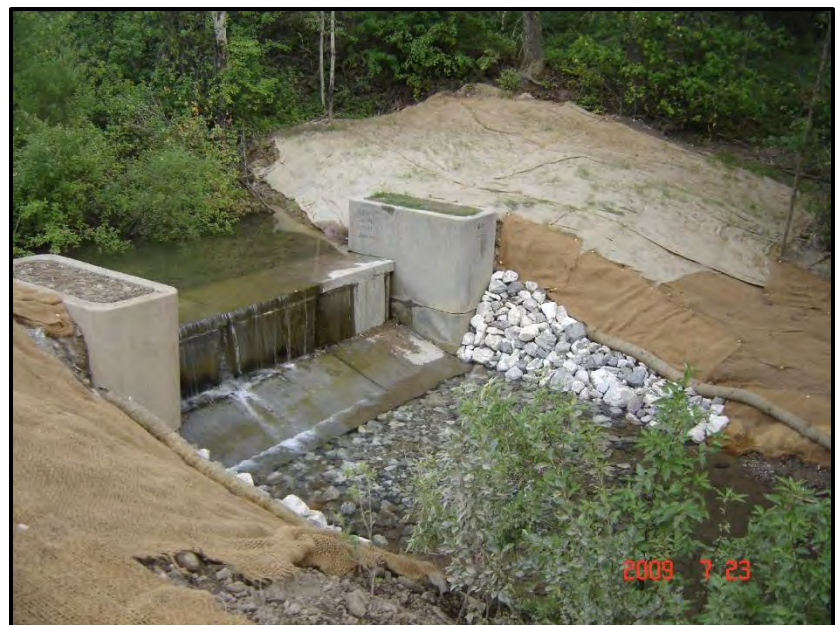
Photo Illustration 2. Fish passage barrier projects constructed on Cottonwood Creek and White Gulch for the purpose of protecting genetically pure westslope cutthroat trout from invasion by non-native fish, including rainbow trout, brown trout and brook trout. The upper photo shows the new fish passage barrier constructed on Cottonwood Creek, a tributary to Holter Reservoir located on FWP’s Beartooth Game Range. The lower photo shows a new fish passage barrier constructed on White Gulch, a tributary to Canyon Ferry Reservoir. The upper photo is courtesy of Allied Engineering. The lower photo is courtesy of Ron Spoon, FWP.
