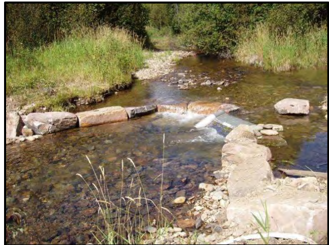
Photo Illustration 4. Fish screens installed on irrigation diversions located on Morrell Creek and Ninemile creeks. Morrell Creek, a tributary to the Clearwater River located near the town of Seeley Lake, supports an important fluvial bull trout population. The Morrell Creek project (upper photograph) involved reducing entrainment into two irrigation canals by installing fish screens, improving upstream fish passage, reducing periodic channel disturbance and enhancing instream flow while continuing to meet the needs of the water user. Ninemile Creek is a tributary to the Clark Fork River located near the community of Ninemile that supports westslope cutthroat trout, rainbow trout, brown trout and mountain whitefish. The Ninemile Creek project involved installation of a coanda style fish screen to prevent entrainment into the irrigation canal and installation of a vortex rock weir to enhance upstream fish passage while meeting the needs of the water user. The lower left photograph shows the Ninemile Creek diversion before project completion. The lower right photograph shows the installed coanda fish screen and vortex rock weir. All photos courtesy of Ladd Knotek, FWP.
