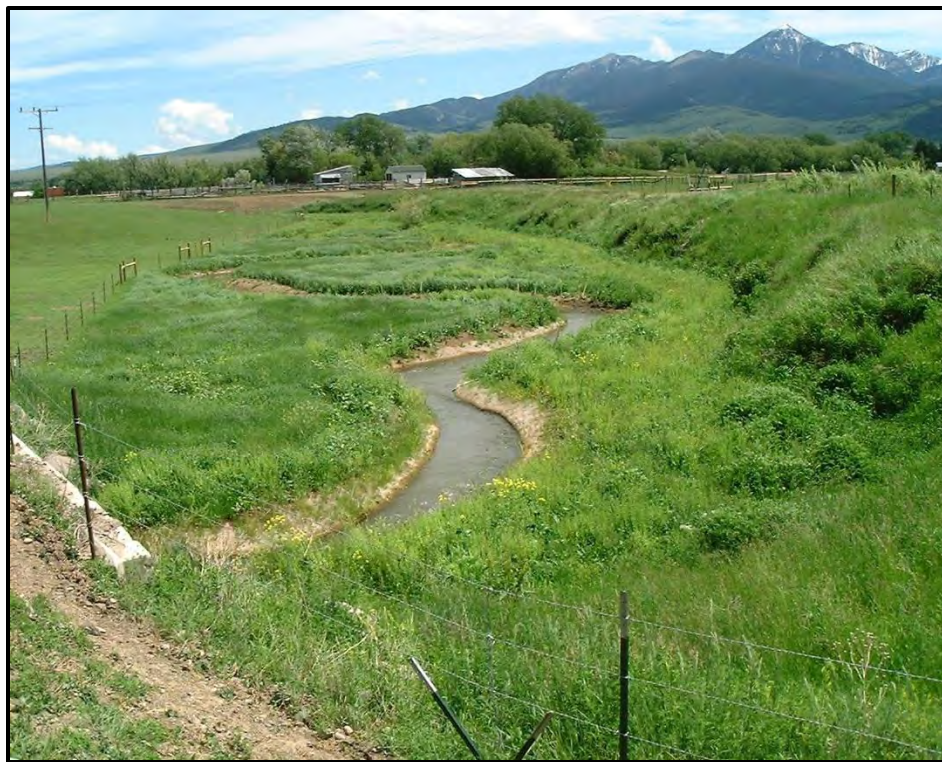
Photo Illustration 5. Channel restoration on Fleshman Creek, a tributary to the Yellowstone River near the town of Livingston. This reach of Fleshman Creek had historically been subjected to channelization and heavy livestock use. This project restored the morphology of 2,400 feet of stream channel and greatly enhanced the floodplain and riparian vegetation while continuing to maintain the agricultural viability of the ranch. The project has benefitted a mixed assemblage of fish including rainbow trout, brown trout, brook trout and Yellowstone cutthroat trout. The upper left photo shows the stream channel prior to restoration. The upper right photo shows the stream channel during construction, including the coir fabric used to form the newly created stream banks. The lower photo shows the restored channel following one growing season with the exclusion of all livestock.
